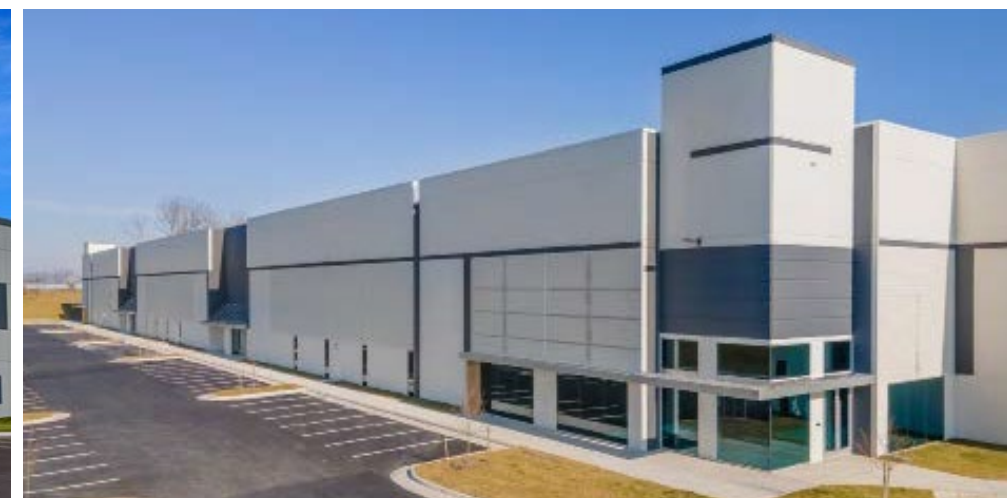
Parkway 66 High Bay Warehouse, Manassas, VA
