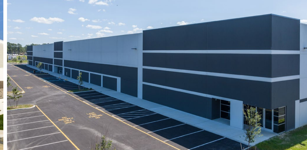
Northlake II 5-Building, 655,000 SF Industrial Park
